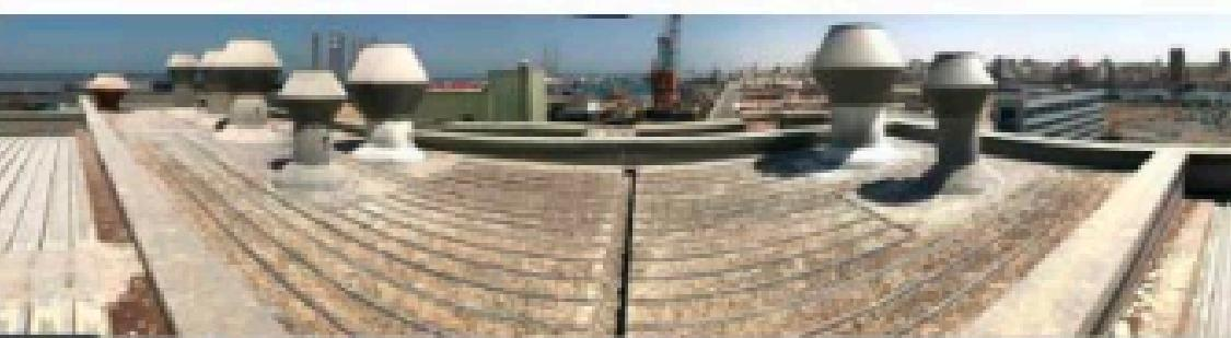
This roof has a Small Valley Gutter and an Eave Gutter at the far end of the roof and 4 downspout in each gutter. The gutter length is around 4.66 meters. However, there is too much Bird Waste on the roof and in the gutters resulting in complete clogging of the drains and water then penetrates from the sheet terminations underneath the sheet and the gutter. Heavy Maintenance is required of this area as well as to replace the gutters since these are also rusted.
