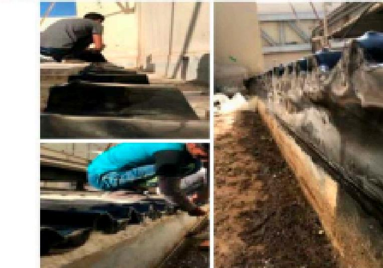
The UNCURED EPDM is a special product being used to prevent leaking of the water from the sheet terminations and gaps. This is being sealed properly at the joint terminations using the German Bonding Adhesive.
